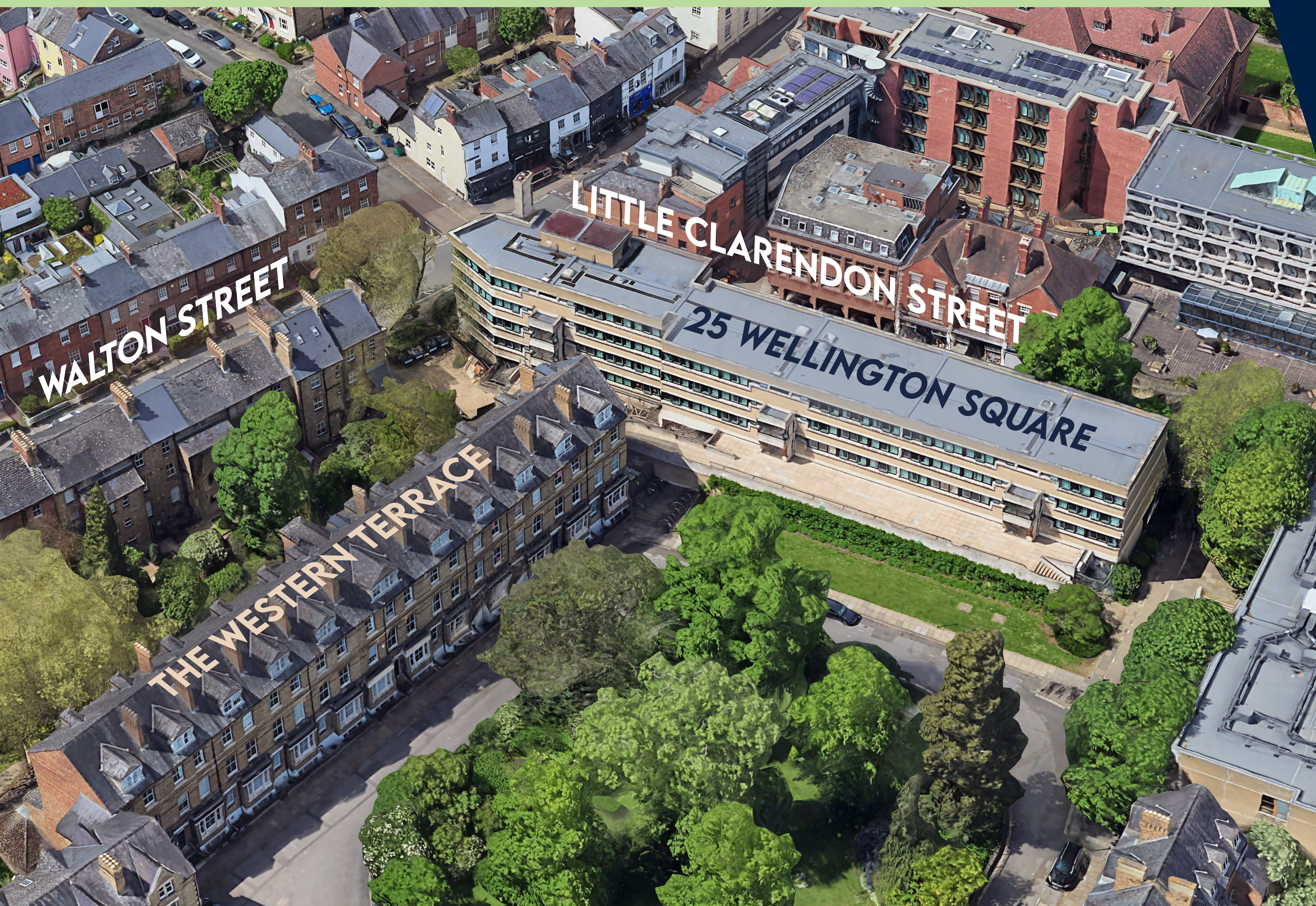
Aerial view of Wellington Square
