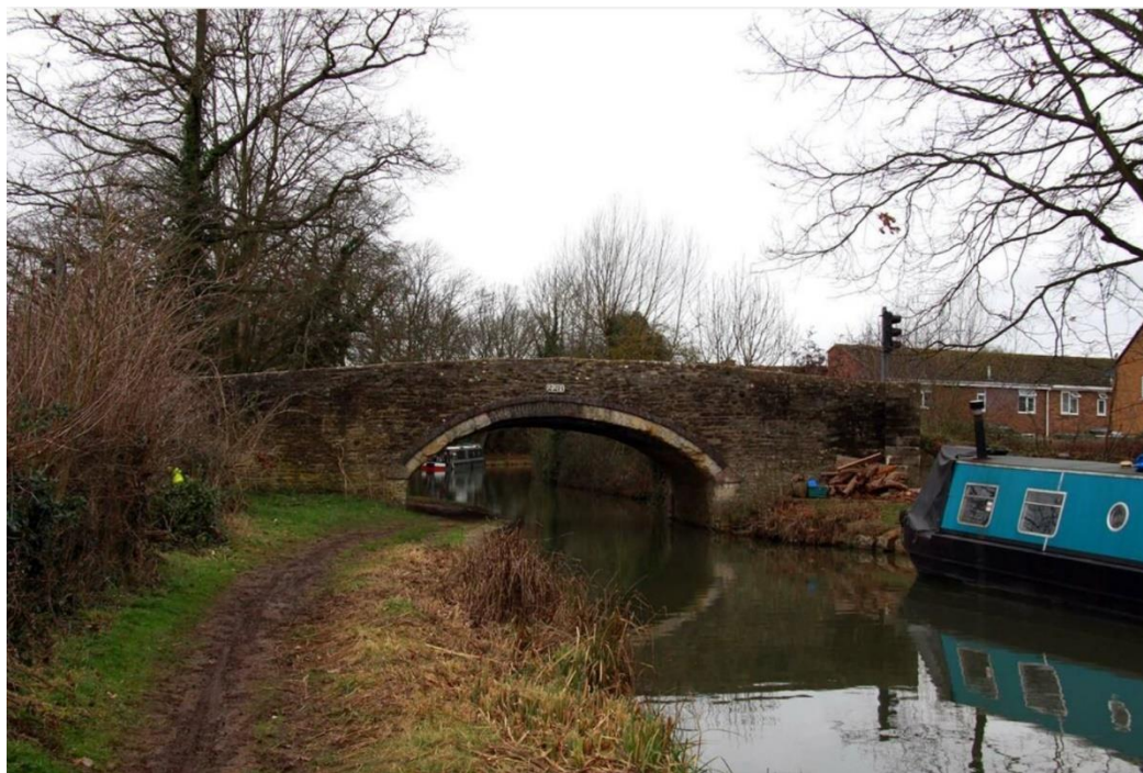
Yarnton Bridge over the Oxford Canal
