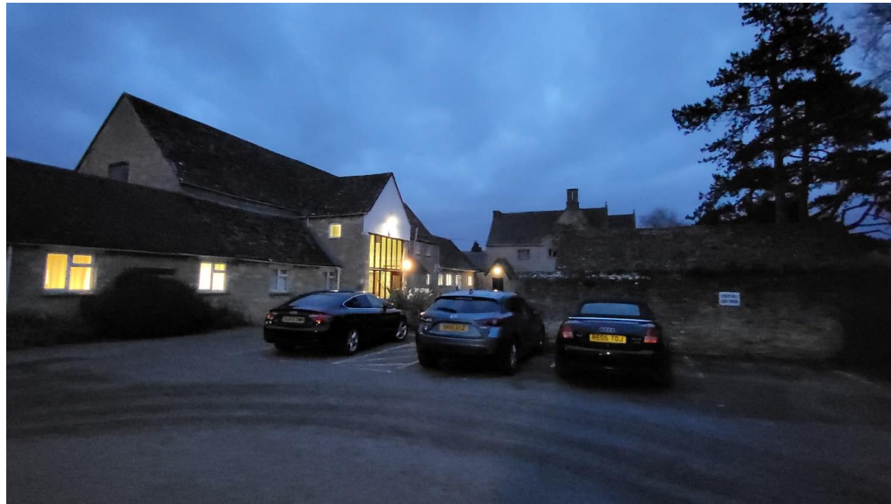
Figure 2.4 – View 2 East – Begbroke farmhouse.
