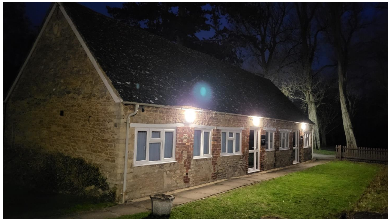
Figure 2.6– View 3, South – Begbroke farmhouse.
