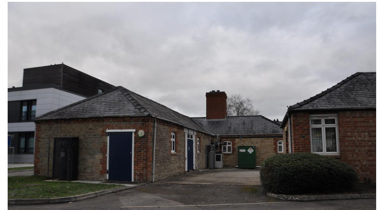
Figure 2.3 – View 1, North – Begbroke farmhouse.
