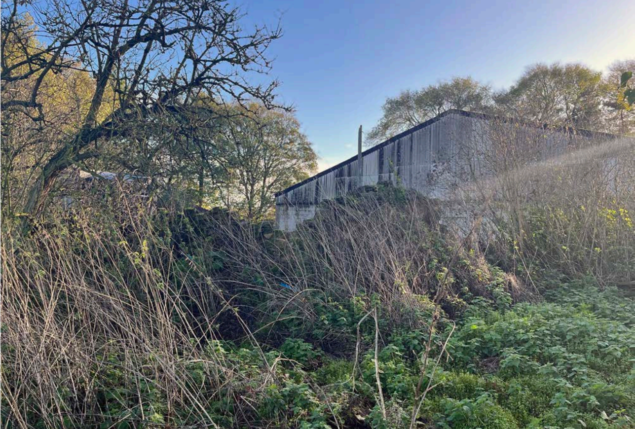
Plate 8: View south. Ruined wall behind agricultural buildings
