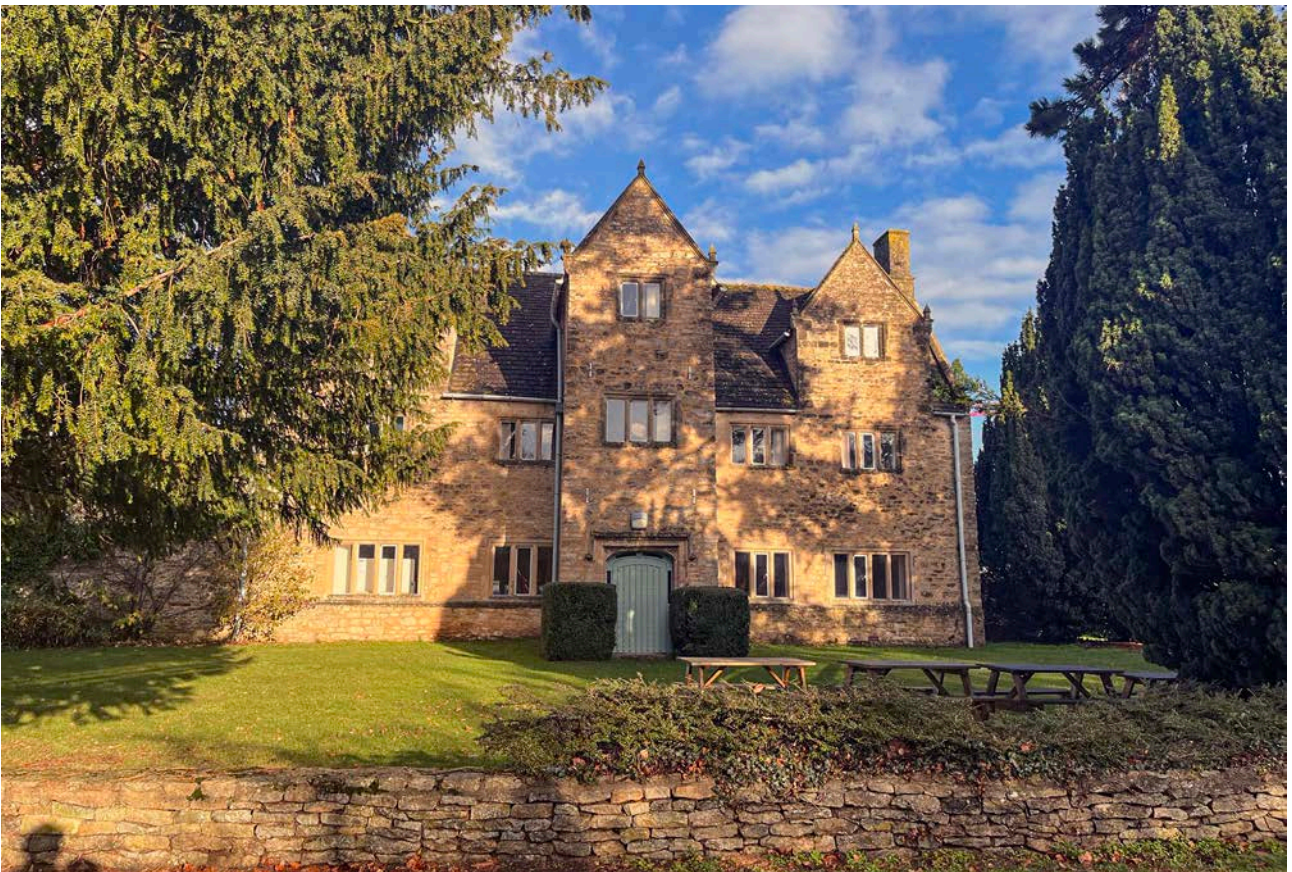
Plate 2: South-facing elevation of Bebroke Hill Farmhouse
