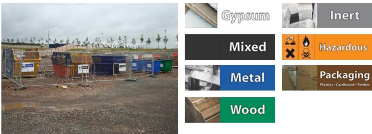
Figure 6—1 Examples of segregation skips on site and waste stream segregation colour coded signage
