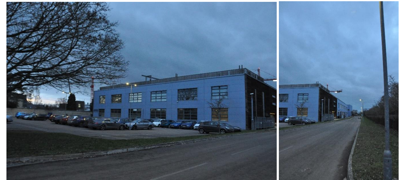
Figure 2.8 – View 5, Northwest – External car park and access roadway.
