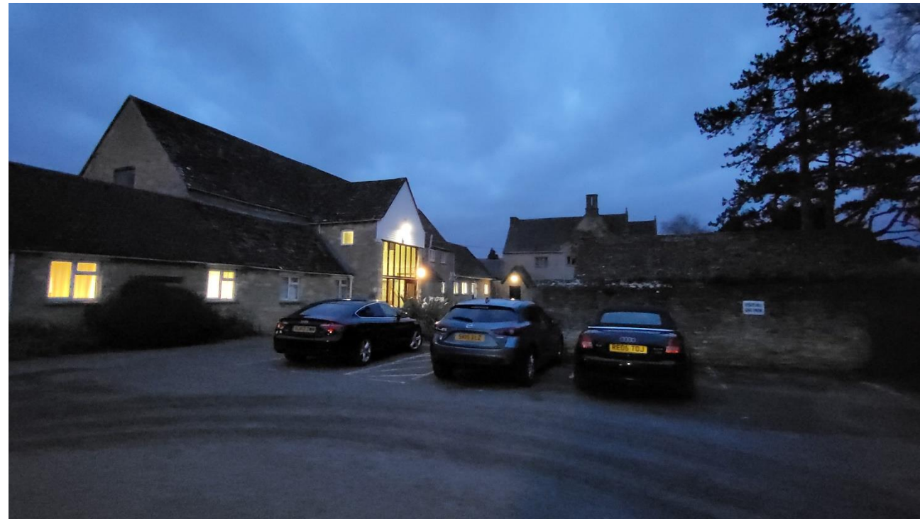
Figure 2.4 – View 2 East – Begbroke farmhouse.
