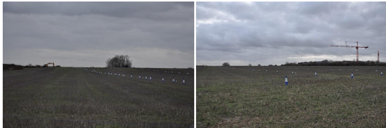
Figure 2.19 – View 16, South and Southwest.
