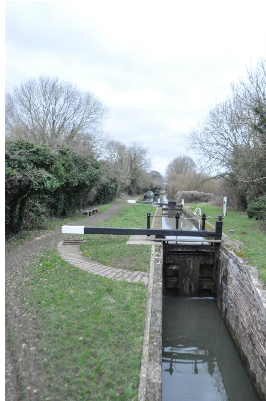
Figure 2.20 – View 18, South – Roundham Lock.
