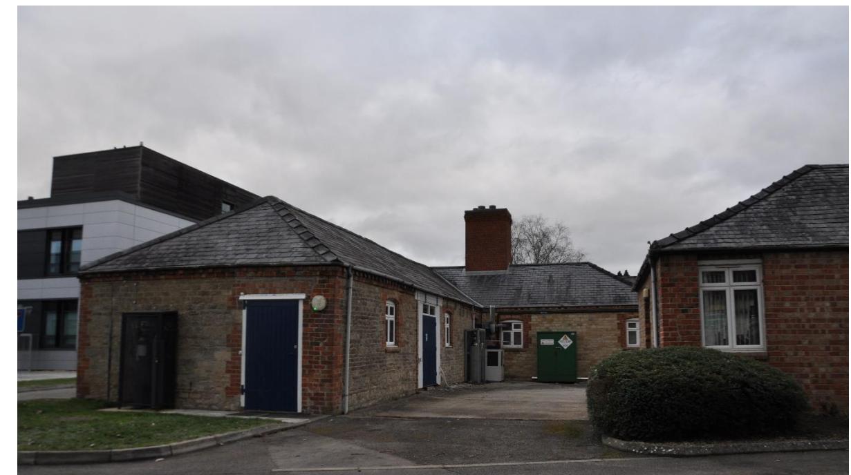
Figure 2.3 – View 1, North – Begbroke farmhouse.
