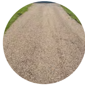
Chip seal asphalt without edging
