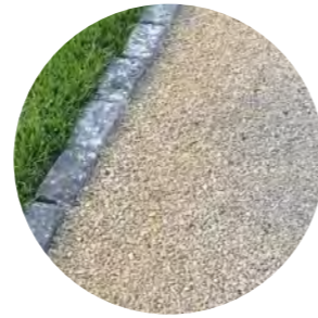
Light aggregate asphalt with cobble edging
