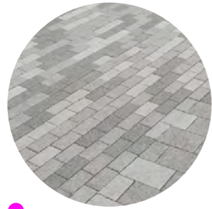
Begbroke Hill Road, Secondary routes, raised crossings and generally all pedestrian spaces/sidewalks: concrete setts with permeable joints. Colour mix differing area to area.
