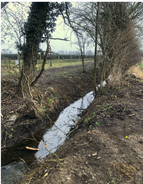
Figure 2.2: Eastern Drainage Ditch system looking downstream in a south-westerly direction. The solar farm is visible on the left bank.
