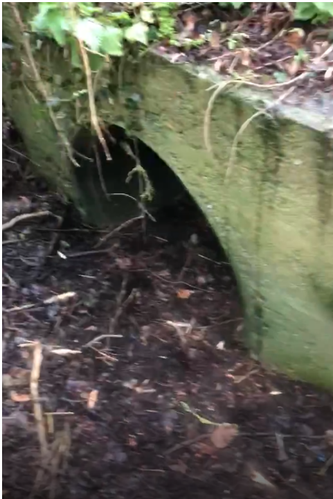
Figure 2.1: Culvert assumed to convey water from the western to eastern ditch along Yarnton/Green Lane
